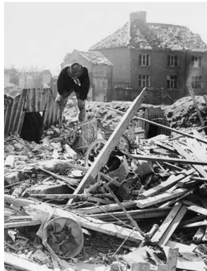
Caption: Inspecting bomb damage, WW2
