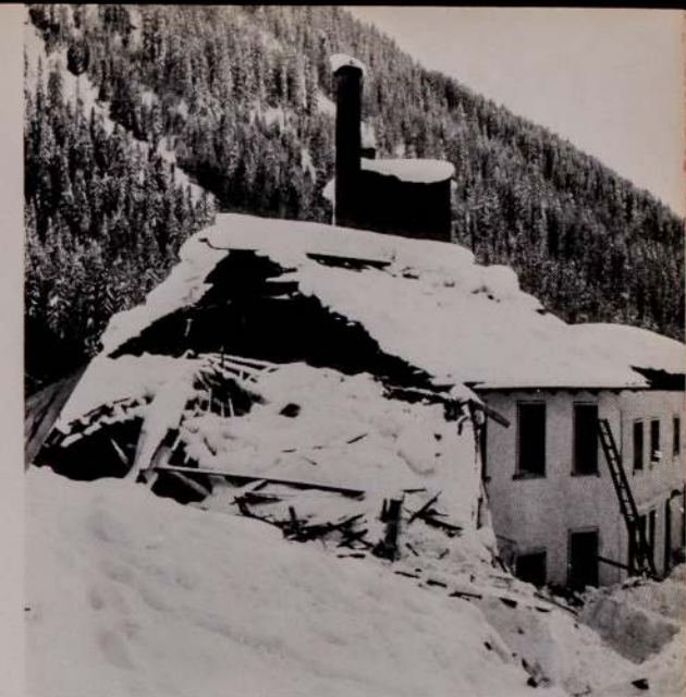
A ruined saw-mill in the Dischma Valley looks as if a bomb has hit it rather than an avalanche.
