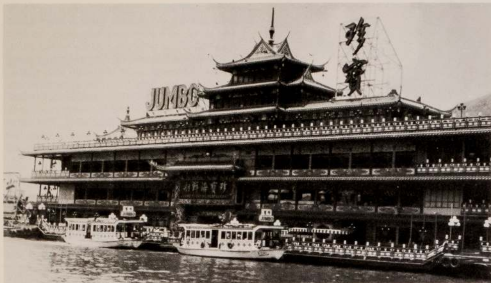
Floating restaurants in Hong Kong Harbour
