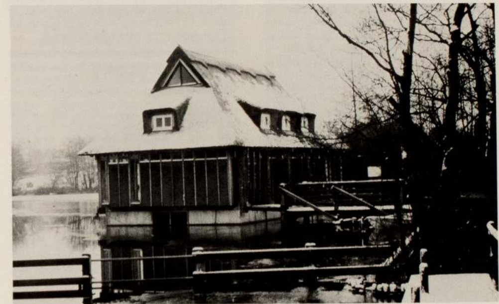
The Broadland Conservation Centre, Ranworth, in winter.
