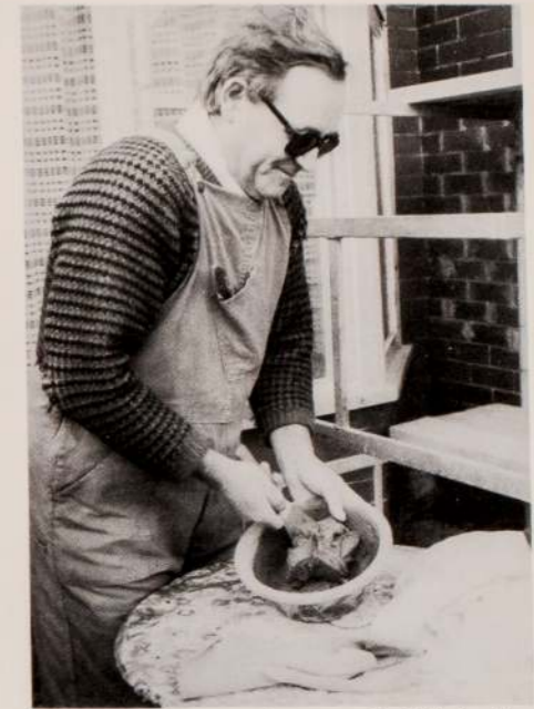
Mixing the sand and cement in Julia's play bucket.
