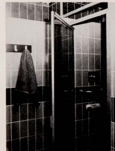
The shower, with door and hand-rail.
