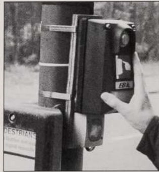
We have also sound-boxes. A tapping sound attracts blind pedestrians to the crossing control button.
