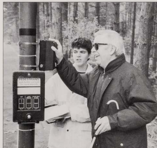
Tracy Savill observes as Terry Walker gets to grips with a tactile crossing guide.
