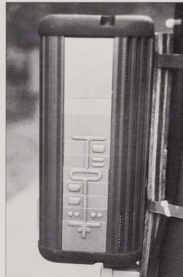
This tactile diagram indicates the presence of an island at the crossing's centre.
