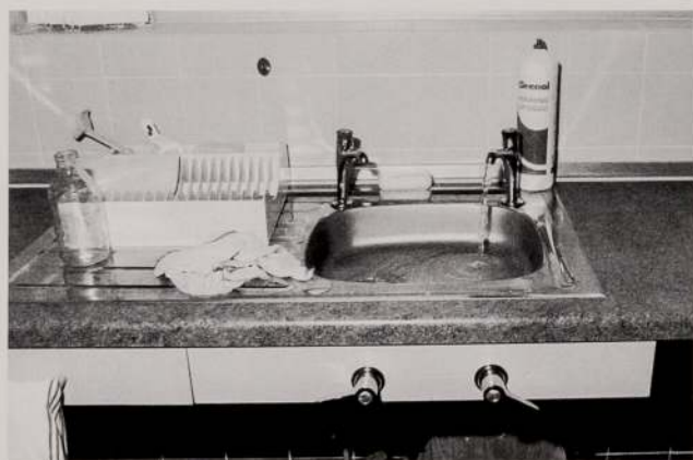
The faucets at the front of this low-level sink unit allow a wheelchair user to draw water with ease.
