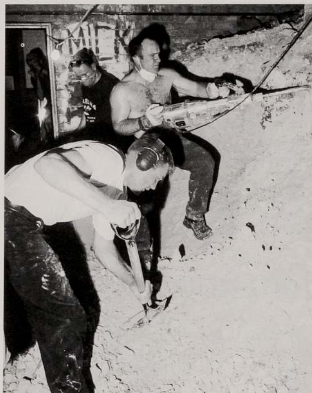
Around 40 tons of chalk was removed by the Sandhurst cadets.
