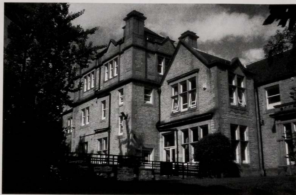
Soon to be St Dunstan's Sheffield - our new training centre.
