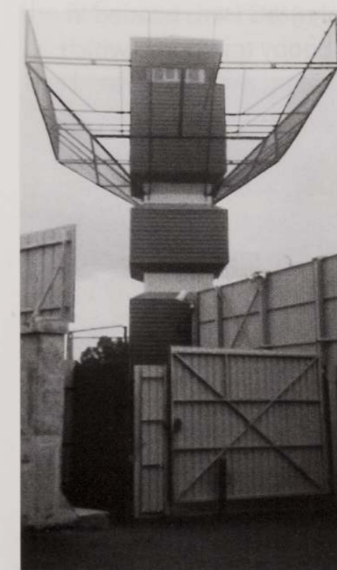
Lookout Block C (also known as The Hump) in Strabane overlooking Lifford.
