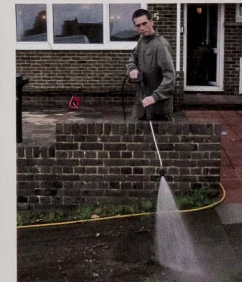
Spray cleaning the path.
