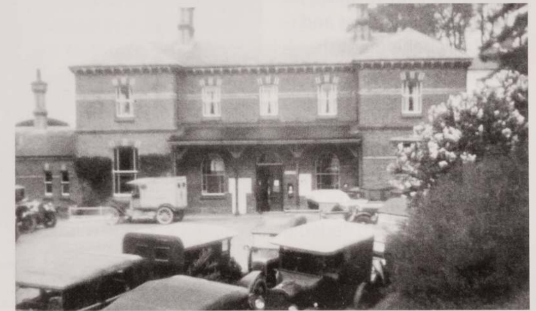
Steyning Railway Station during the General Strike.
