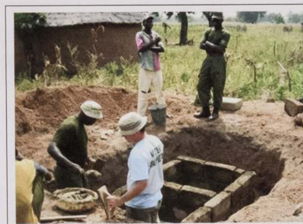
Picture: Building latrines.
