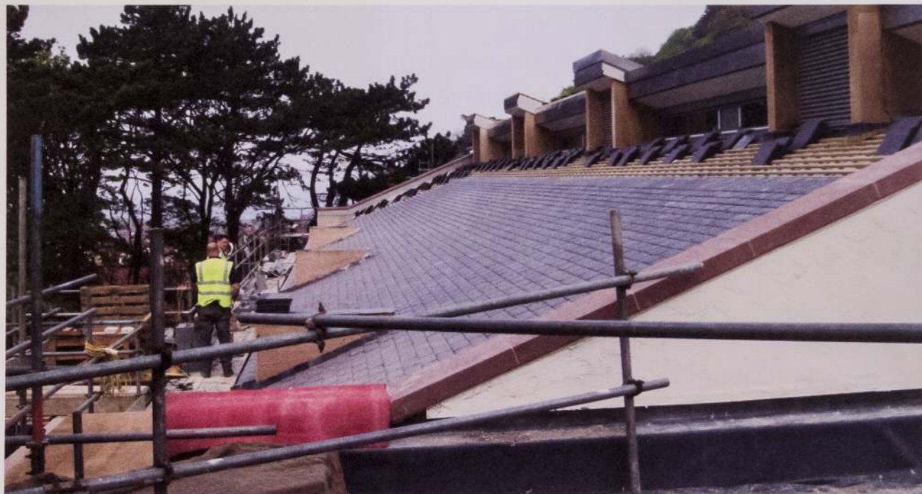
Picture: Extension roof with the majority of slates fitted.
