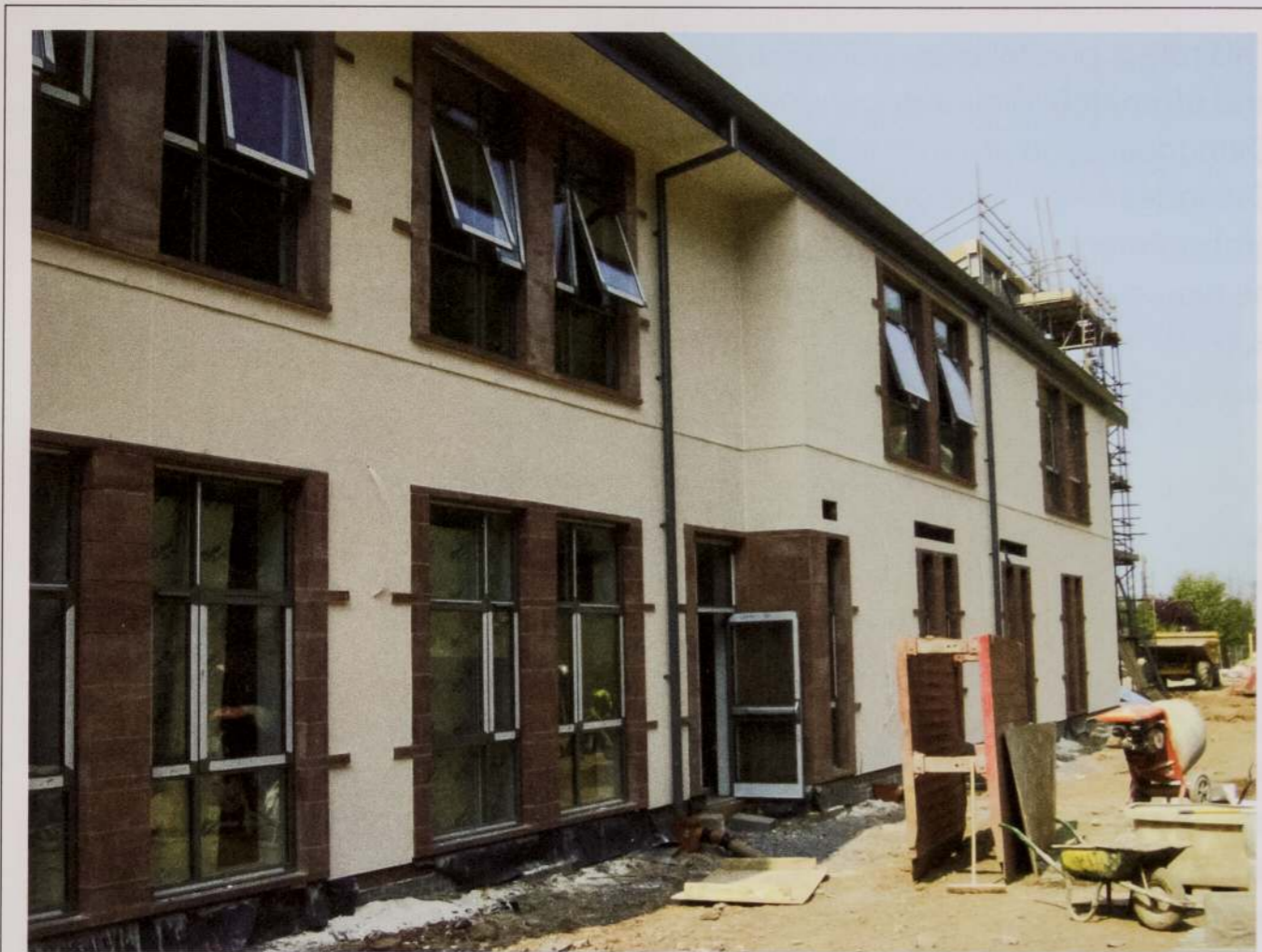
Picture: Work in Progress - The extension at Llandudno.
