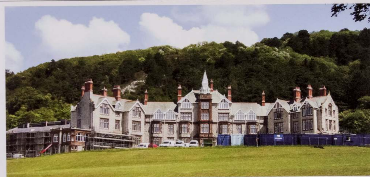
Picture: Work progresses at the Llandudno Centre.
