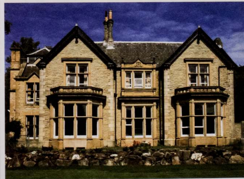
Picture: The Sheffield centre is another historic building that was originally the home of a cutlery manufacturer and his family.
