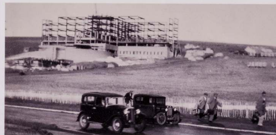
Picture: The Brighton centre under construction in 1937.
